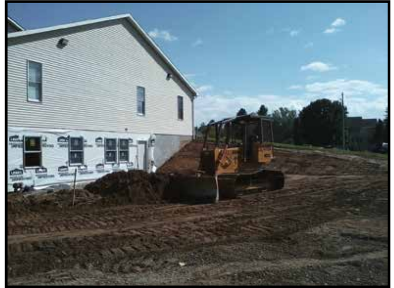
Site work and backfilling around the new addition.
